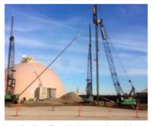
length piles, Bermingham reduced the total pile installation by a month. See the photo above of Bermingham VTL System lofting a 100 foot pile.
